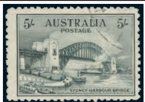
1377. ○ 132, Five Shilling Sydney Bridge, F+ ..... 275.00
