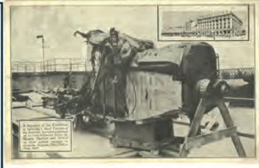
The damaged Sopwith Atlantic was used and put on display in Selfridge's Roof Garden, London. 1. while practising for the Aerial Derby at Hendon, Harry Hawker's plane pitched into the earth at low level only. The precise cause of the crash was never determined. There was suggestion that Hawker had suffered a spasm, or that the carburettor float had come loose and caused a fire.
